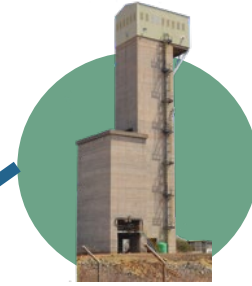
SELEBI UNDERGROUND MINE
